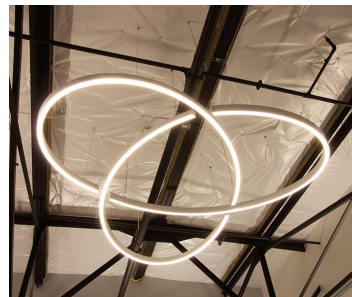
Tangent Down with custom curvatures in plan, terminating in custom mitered ends, which compliment the intersecting radii
